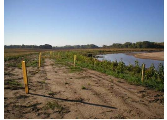
Once the structure sequence is determined, their heights and widths are selected based on water depth and channel materials. Our stream design team has developed efficient methods for estimating rock quantities and the amount of soil to be moved in order to reshape the vertical stream banks as well as accurately estimate construction equipment time.
