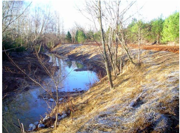
Goodwin Creek – After Construction – Looking Downstream –
