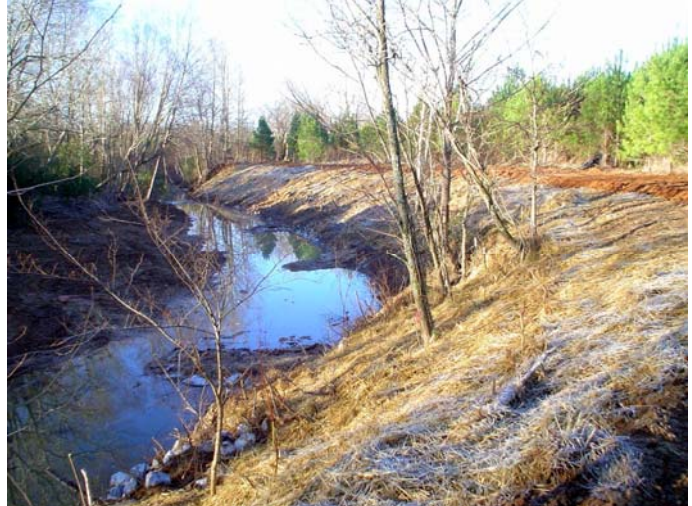
Goodwin Creek – After Construction – Looking Downstream
