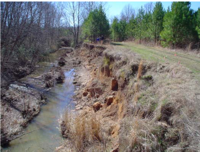
Goodwin Creek – Before Construction – Looking Downstream
