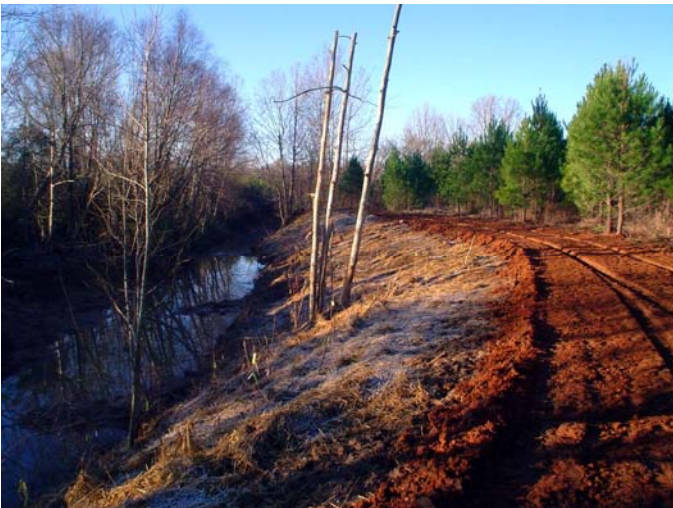
Goodwin Creek – After Construction – Looking Downstream – Transplanted Sycamores in the middle bank.
