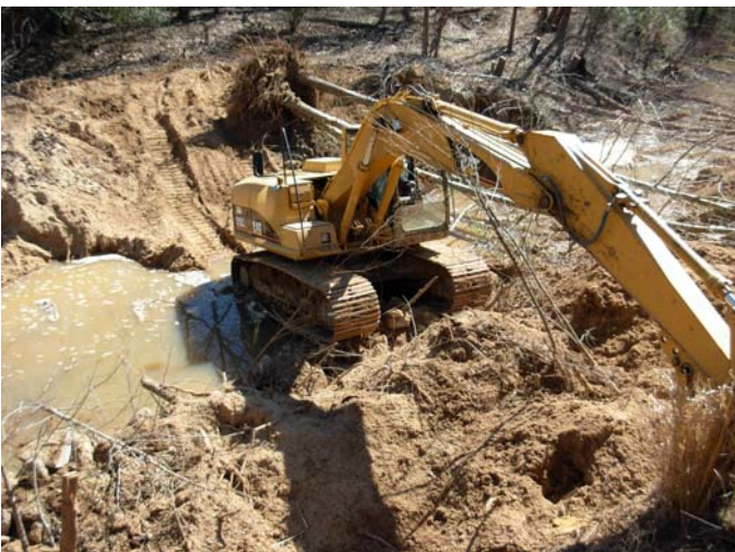
Goodwin Creek – During Construction
