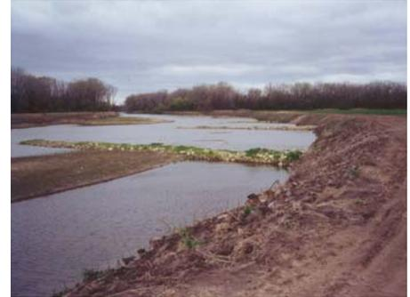
Once the structure sequence is determined, their heights and widths are selected based on water depth and channel materials. Our stream design team has developed effective and efficient methods for estimating rock quantities and the amount of soil to be moved in order to reshape the vertical stream banks as well as accurately estimate construction equipment time.
